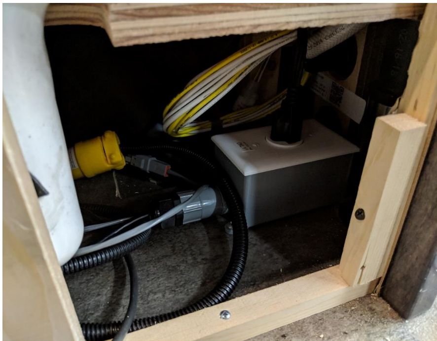
Figure 39: Installed heater box with wires placed inside access panel
